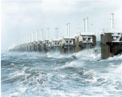
Safety, protection against flooding
