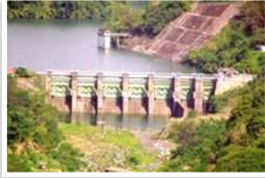
IPO DAM (MWSS)
